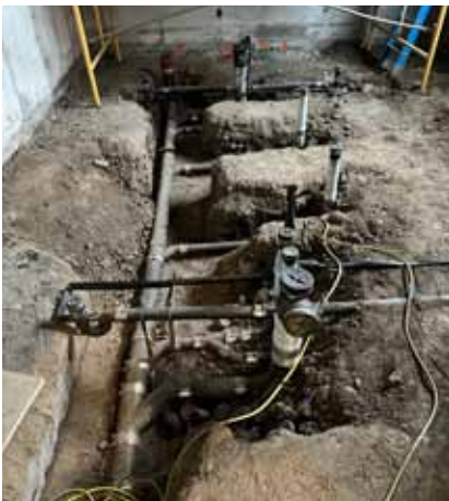
THE NEW ROUGH PLUMBING GETTING INSTALLED IN THE OLD BOILER ROOM.
